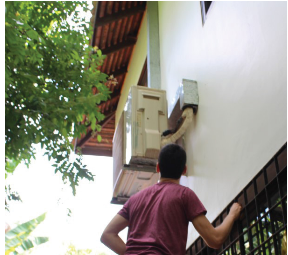
AC outdoor unit on the façade correctly protected by an overhang
